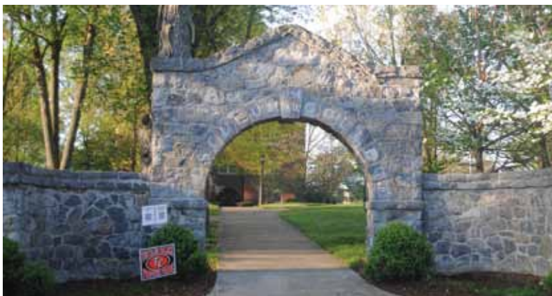
The restoration work was completed in time for the Arch to welcome visitors to campus during the Old Oak Festival.
