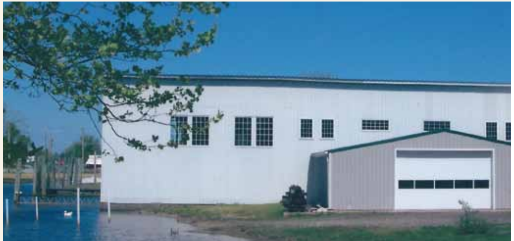
The shipyard now has an attractive covered area for boat launches.
